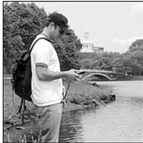
Dave Kaplan, a CRWA watershed scientist, stands on top of eroding bank of the Charles River in Allston, where at least two acres of parkland have been lost to riverbank erosion.
