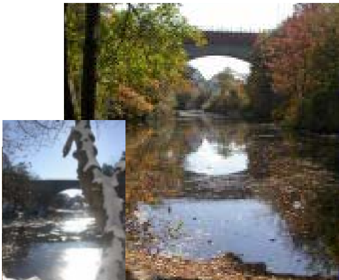
Winter scene at Hemlock Gorge Reservation looking at Echo Bridge
