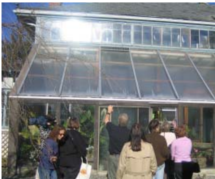
An enthusiastic group enjoyed an 'Urban Ark' Seminar and Tour. This passive solar greenhouse was added to a 6,000 square foot Newton house and heats the house most of the heating season with the help of a fan powered by a photovoltaic solar panel that distributes the warm air through connecting second story windows and doors. Money is saved using waste water for irrigation.
